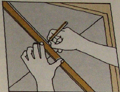
3 Mark diagonal lines on the existing pane with a crayon or china-marking pencil, to find the centre-point
