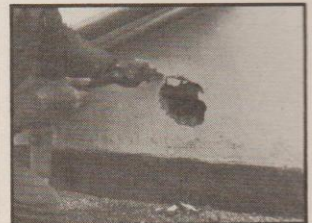
3: Chopping from the outside of the house to complete the hole
