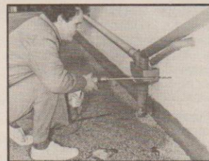
1: Using a special long masonry bit to drill right through the wall – to mark the centre of circular fans or the four corners of square ones
