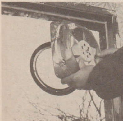
14. With the rim fixed in position, the body of the fan is slipped into place
