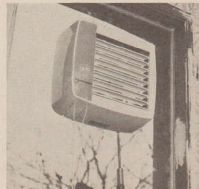
16. The internal fan fascia is secured to the main body with screws provided
