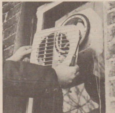
15. Once the fan's body is secured to the rim, the outside casing is mounted
