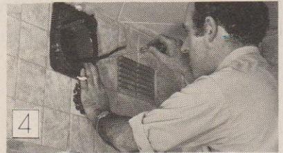
4 Mount inner and outer clamp plates.
