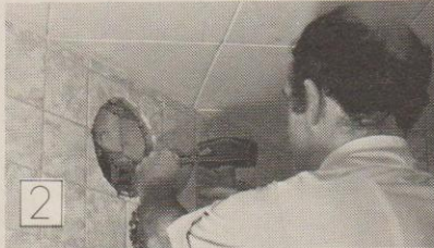
2 Open up the hole through the wall.
