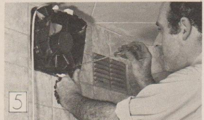
5 Fit fan unit and block up redundant vent.
