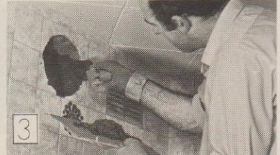
3 In solid walls, line the hole with mortar.
