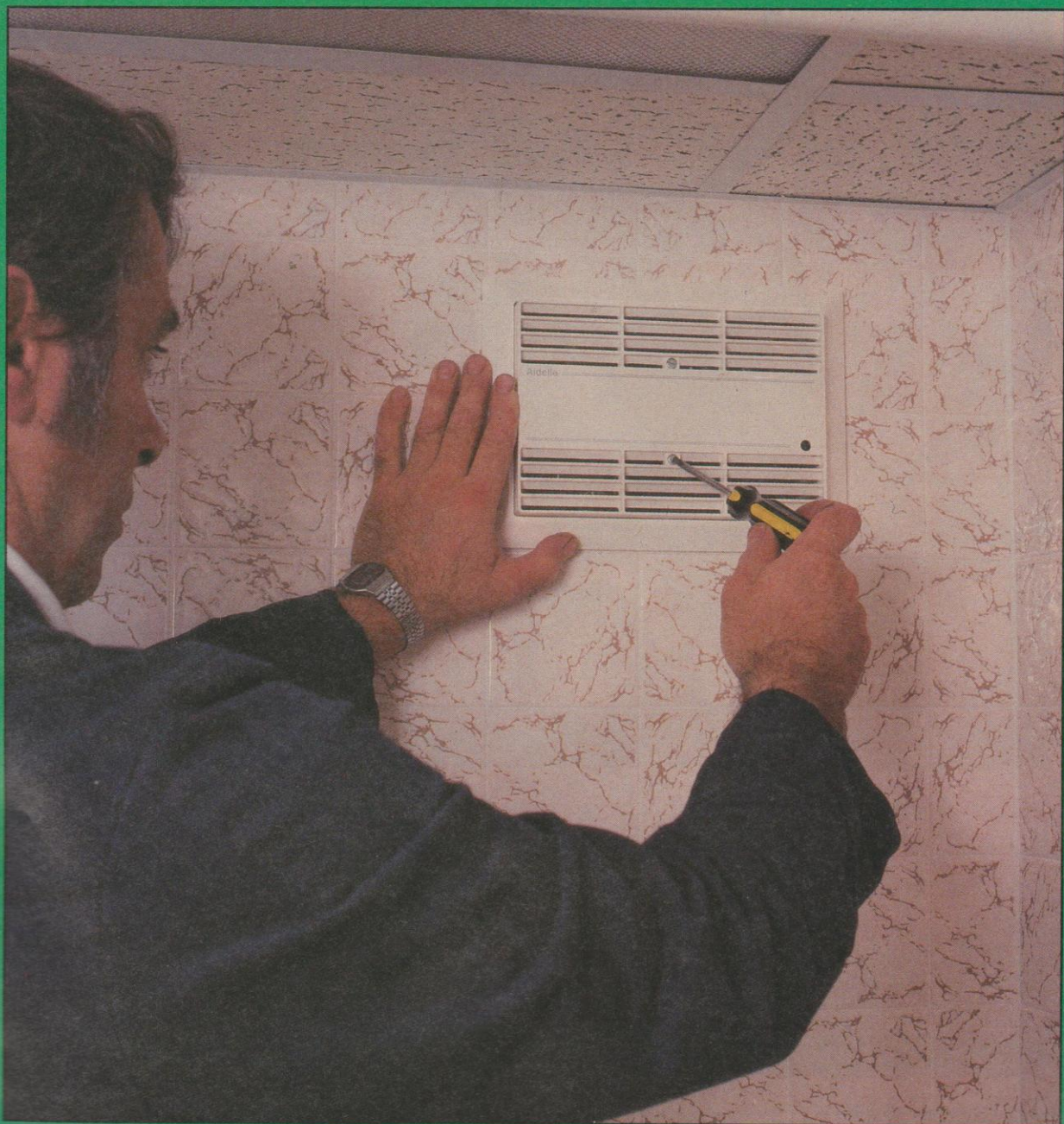
Ensuring the sweet smell of success: installing the Aidelle Loovent 07.
