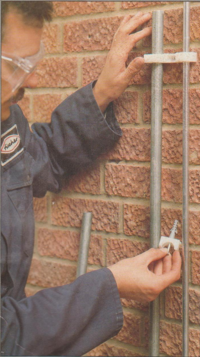
One for the fixture list — The SCH Saddle and S Plug from Fischer Fixings.
