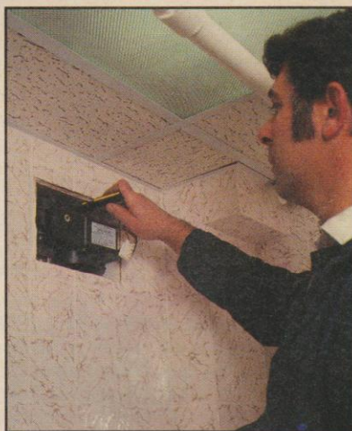
Once the motor is fitted, the grille is fixed for the final finish.
