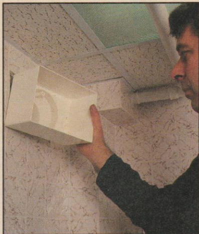
The wallfan housing is fitted into the wall with the motor following after.
