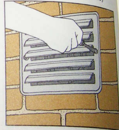
11 Place the outer grille over the flange and screw it home. Connect cable to terminals and switch on
