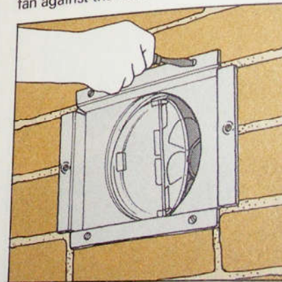
10 Outside the house, position outer grille sleeve. Drill holes at top and bottom, and plug and screw to wall
