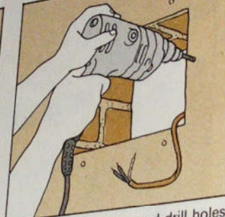
5 Remove fan section and drill holes for fixing screws provided with fan. Fit wall plugs in holes (see p. 683)
